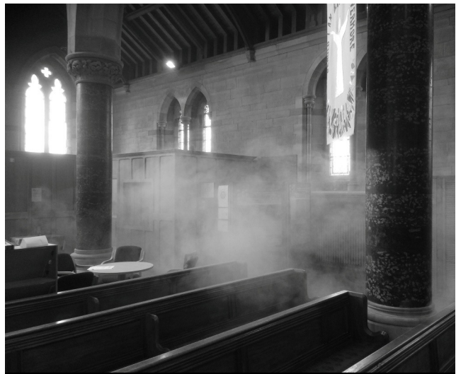
ABOVE: A scene reminiscent of Isaiah 6:4 "and the house was filled with smoke". Sadly, no-one was seeing the Lord..... just some repair work to the tiled floors at St Paul's. Removing stubborn masonry required machine tools and created a large cloud of dust!
